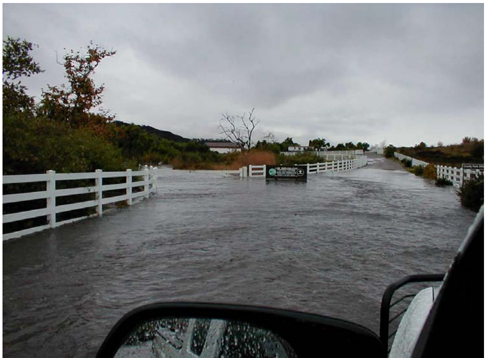
Flooding around the historic ranch house in Peñasquitos Canyon Preserve during the October rains. Photo provided by County Rangers.
