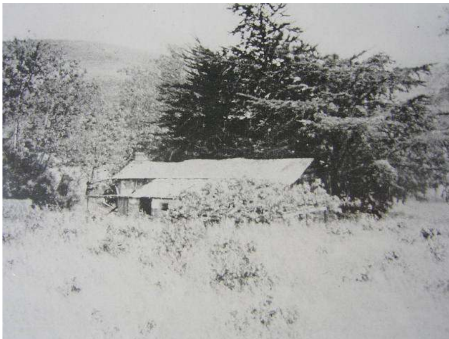
Bovet adobe in a dilapidated condition with only 1/2 the roof — notice the close cropped grass from the presence of cattle and a wall with a passage knocked thru it.
