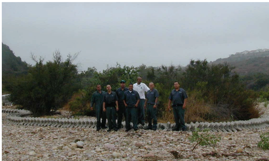
Urban Corps crew pose in front of Ajacks, erosion control structures made of concrete. The crew worked with Mike Kelly to install these in 90 F temperatures. Hard work! Although made of concrete, heavy floodwaters busted through the concrete and swept away part of this terrace with its Monardella plants.
