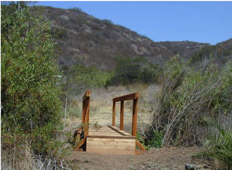
This new bridge crossing Luzardi Creek makes a trail connection between the north and south sides of the creek, a few hundred yards west of where the creek and trail pass under Camino del Sur. Luzardi Creek is an undiscovered treasure of the newly expanded Black Mountain Open Space Park. Visit www.penasquitos.org for a .pdf map of the park! Photo by Mike Kelly.
