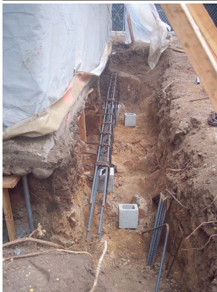
Wing C during restoration. Water damage to the old foundation required the installation of new drainage, reinforcement of the old foundation, and lots more restoration work. Photo by Autumn Acker.
